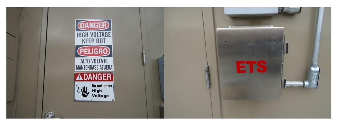
TPSS A-4 side access doors with additional warning signs. Note ETS Emergency Traction Power Shutdown box with reflective "ETS" decal lettering.
