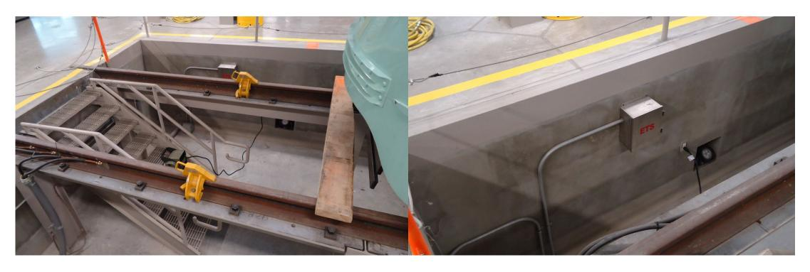
Service bay had wheel blocks installed as soon as the first vehicle has arrived and it's stop position had been determined and installed. Pits have round LED lighting fixtures for better work light focusing. ETS (Emergency Traction Shutdown) boxes are labeled with reflective lettering.
