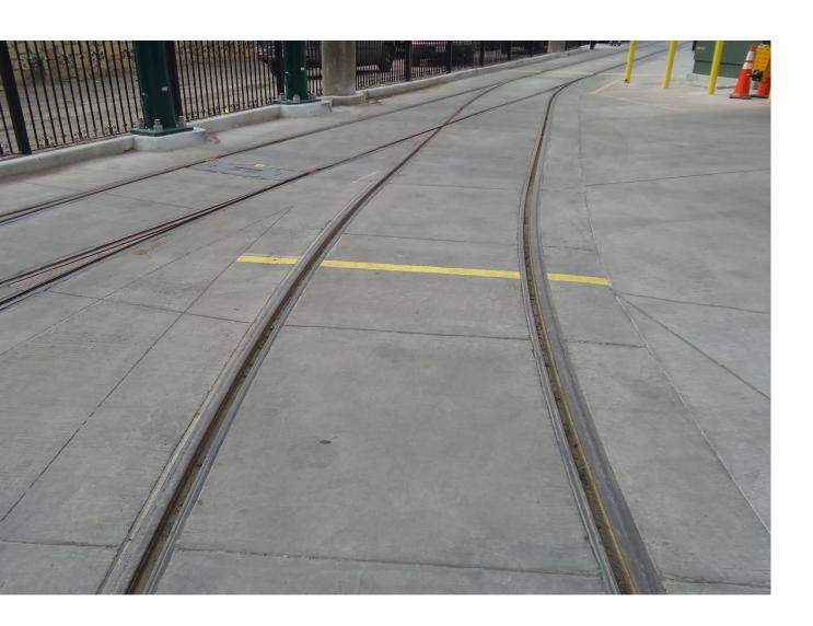
Yard apron features track fouling marks that are painted with highly reflective yellow paint which is easy to see in low light conditions.
