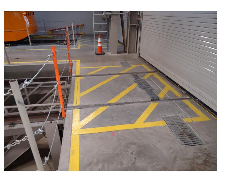
A safe zone to allow a tow vehicle driver the ability to gauge how much room they have to maneuver when pushing/pulling a streetcar in or out of the MSF Bay-1.
