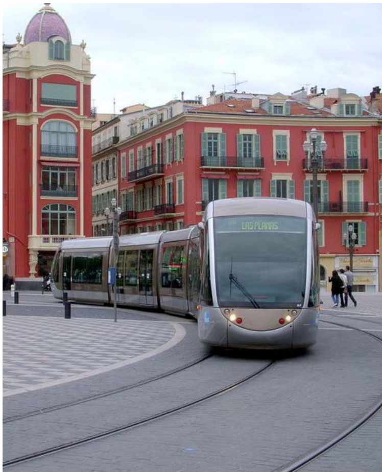
Nice, France - short off-wire segments using onboard energy storage. Opened 2007
